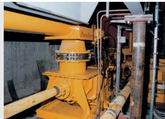
Below: The solids pump KOS 540 conveys over 80 m into the incinerator of the refuse power station at Vestvorbraending, Copenhagen, Denmark
